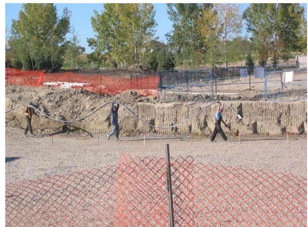
Figure 4. U-tube ready for insertion into borehole
