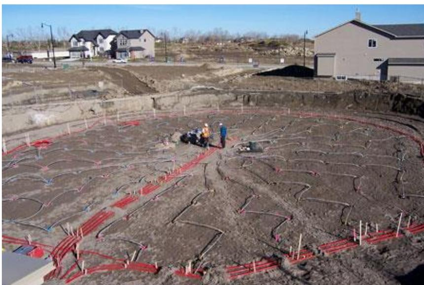
Figure 5. U-tubes connected into 24 near-radial strings and into 4 circuits
