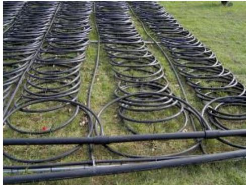
Figure 17: Closed System<sup>35</sup>
