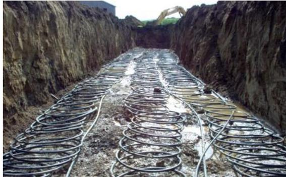
Figure 18: Geothermal Heat Pump - Horizontal Trenches<sup>36</sup>
