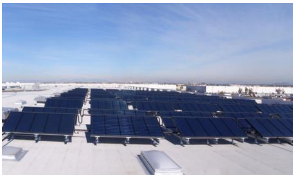
Fig. 13: Solar thermal process plant- hot water production used in the beverage industry (source: SOLID GmbH, Austria)
